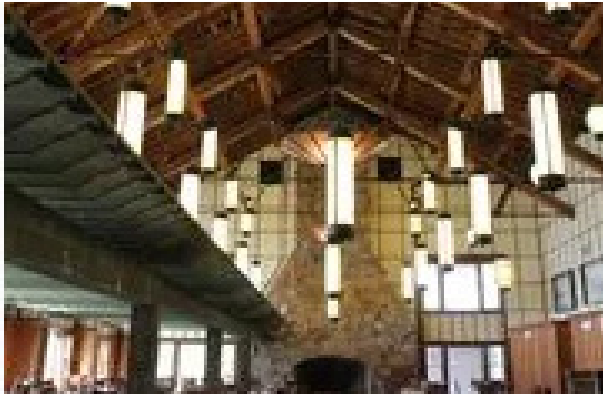
The Ptarmigan Dining Room had a low drop ceiling installed in the late 50's. During the rehabilitation, the drop ceiling was removed, the fireplace was reinforced and a pergola was installed with the same color and style of the original. (Photo: Tribune Photo/Sarah Dettmer)
